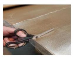
Installation of the detection mesh, instead of the mica sliding layer, easy to cut
